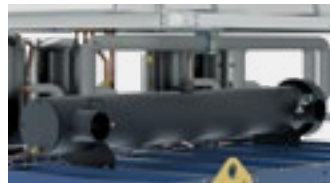
Shell and tube evaporator.
